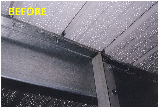
Condensation "rain" prior to Grafo-Therm application
