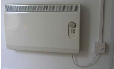
2kW wall mounted convector heater
