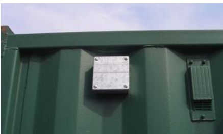
External connection box ready for on-site connection by qualified electrician
